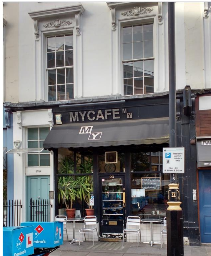
No. 93 Charlwood Street
